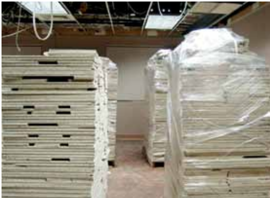
Demolished ceiling tiles are collected for recycling
